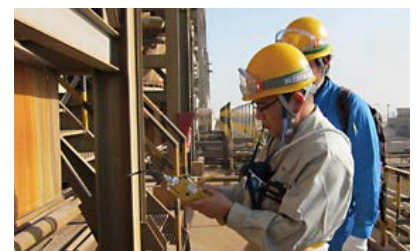
Dammam 2nd Industrial City Field Survey
