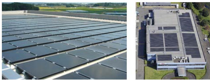
Solar panels at the Sekijyo Plant of Fujitsu Telecom Networks Limited
