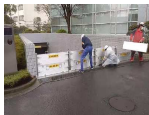
(a) Removable watertight panels
