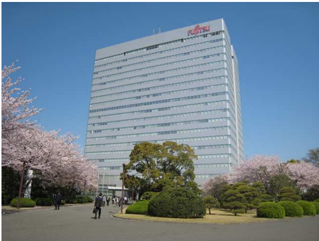
Exterior of Kawasaki Plant
