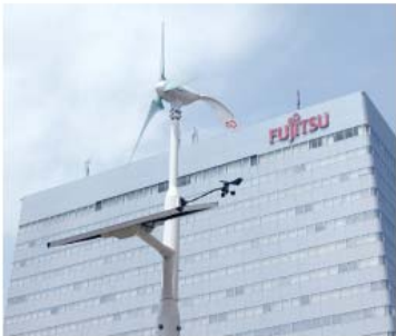
Hybrid Electric Power Generation System
