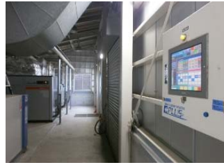
Saving energy activity with combination of compressors with inverter and its demand controller (SHINANO FUJITSU)
