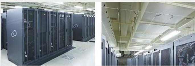
In the Cloud Center, a few optical fibers snake along the ceiling at 50 cm intervals, runs around the fronts and backs of server racks and even under the floor before it connects to the measurement device.
