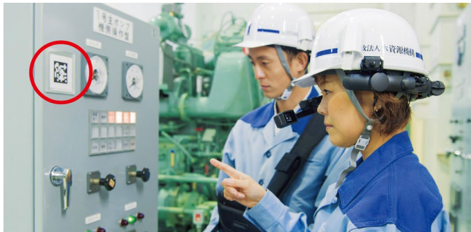
Checking AR-marker-linked work procedures
