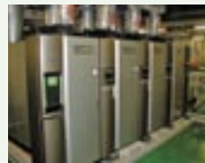
Arai Plant Boiler Installation
