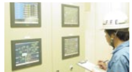
The Management Room at the Akiruno Technology Center
