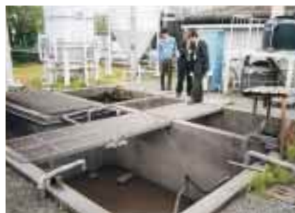
A facility management survey of Fujitsu VLSI's wastewater treatment facility
