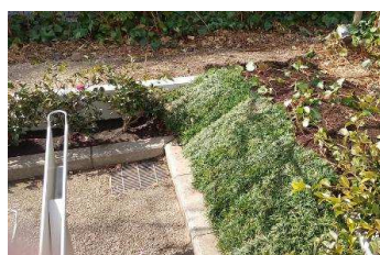
(a) Retaining walls and embankments
