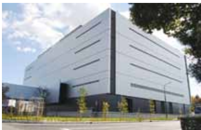
The new annex of Fujitsu's Tatebayashi System Center
