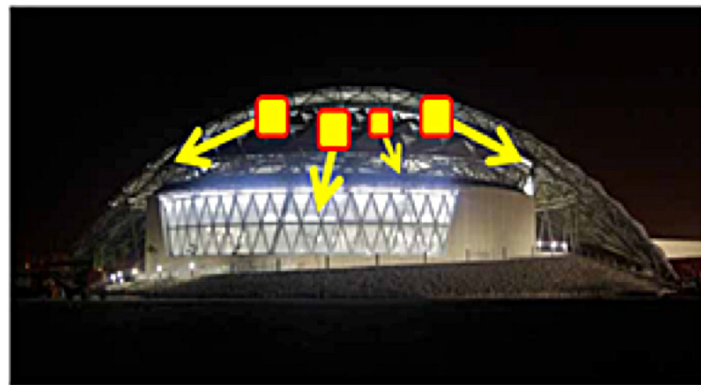
(a) Ceiling Deployment
