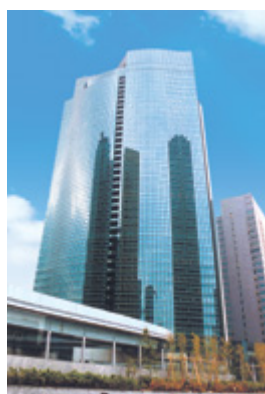
Pic.1 : Fujitsu headquarters, Shiodome City Center.
