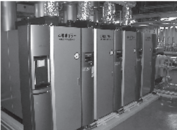
Figure 5 Reduction of CO 2 emissions by switching boiler fuels (Arai Plant, Shinko Electric Industries Co., Ltd.).
