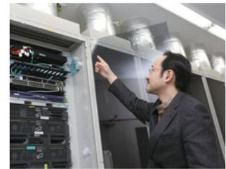
Special ducts that supply cooled air directly within racks and improve server cooling efficiency
