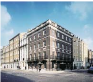
A view of head office.
