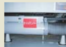
Seismic isolation device (oil damper)
