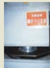
Seismic isolation device (rigid slider support)
