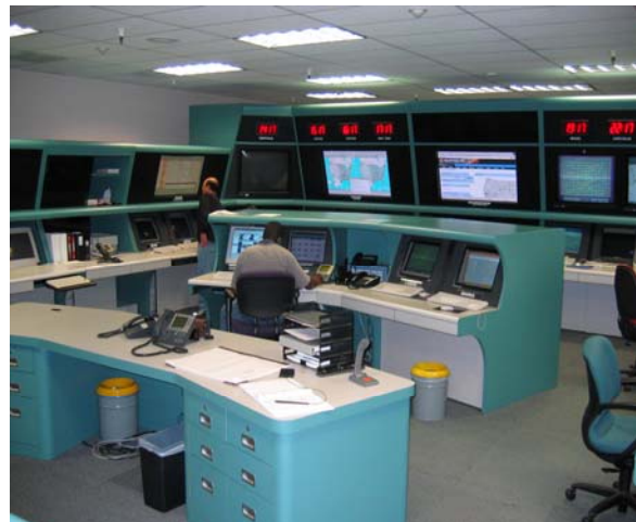
Fujitsu Network Operation Centre (NOC)
