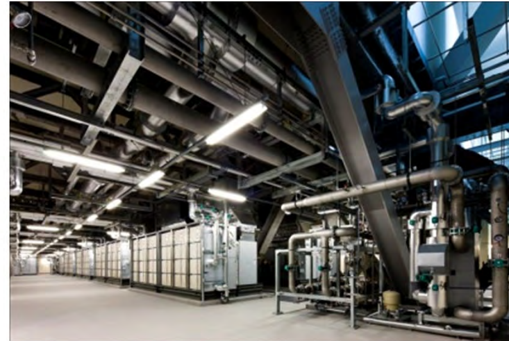
Air Handling Units (Computer building 2F)
