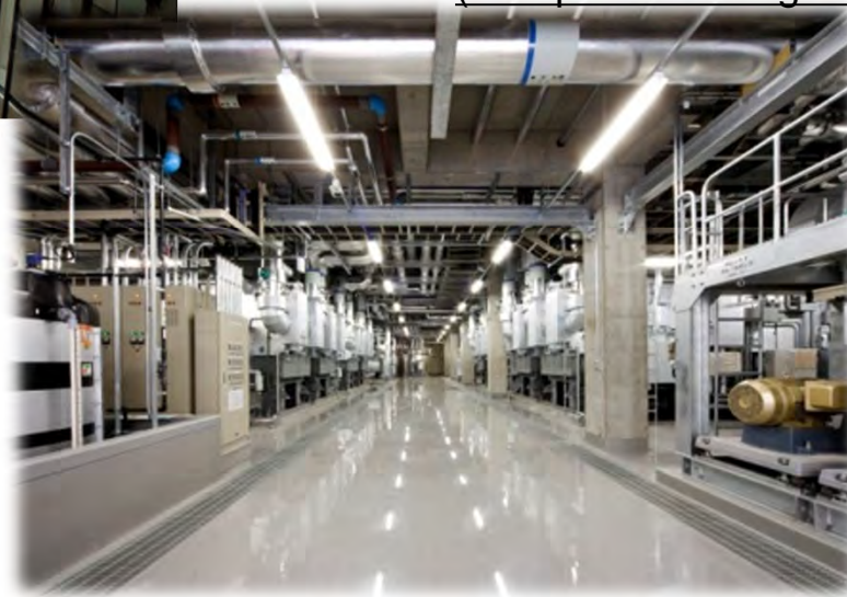
Power Supply and Cooling Unit Building Centrifugal chillers
