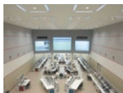
The Integrated Control Room of Tatebayashi System Center
